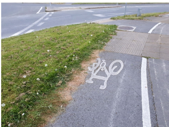
Photo (below): Weed encroachment on cycle way and footpaths (near Naas Road Roundabout) - (UD17)
